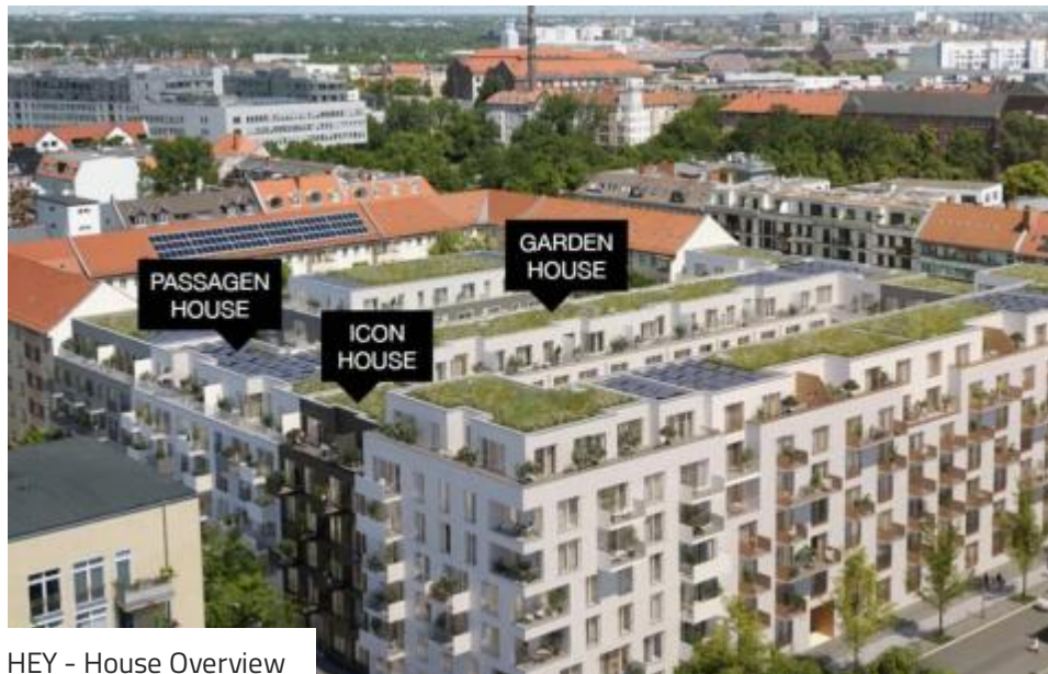
HEY - House Overview
